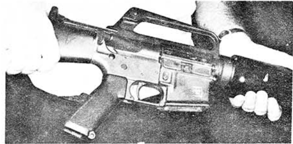
Step 2. Hold Charging Handle Back and Inspect Chamber.
