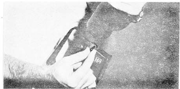
Step 4. Pull Pivot Pin Out to Detent.
