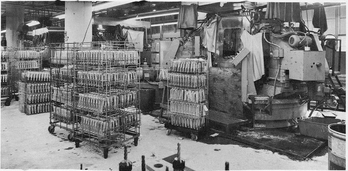
Figure 9-9. | M16 Upper Receiver Machining Area
